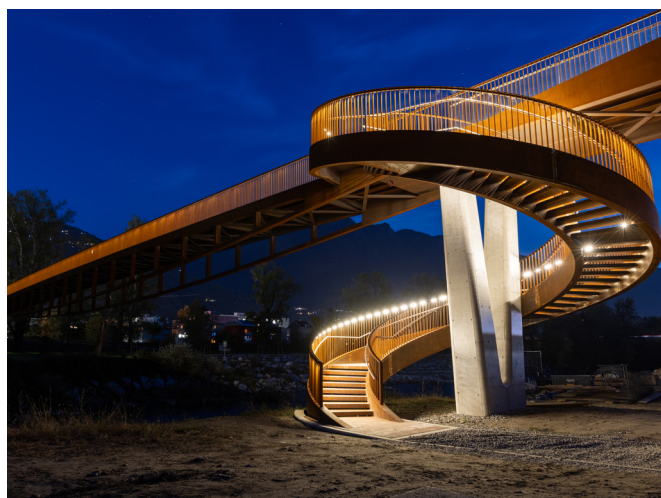
LaneLED WALL, Passerella Torretta Bellinzona
